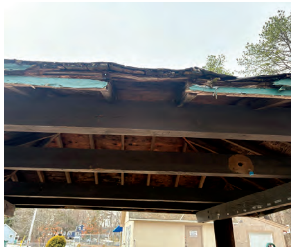
Picnic Pavillion before repairs.
