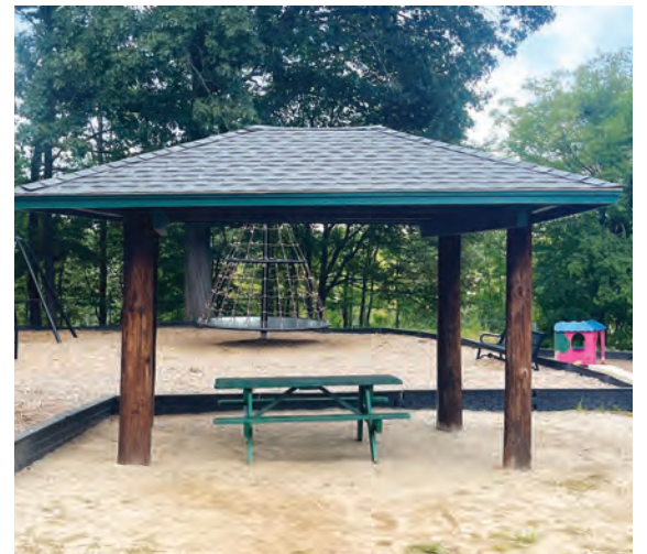
Picnic Pavillion after repairs.
