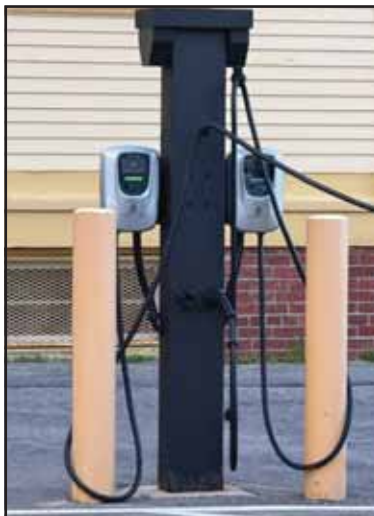
CHARGING STATIONS TOWN HALL No bids, managed by Town Admin. Orlando Pacheco. Required Changes. Contractor: Inovis TOTAL PROJECT COST: $77,524
