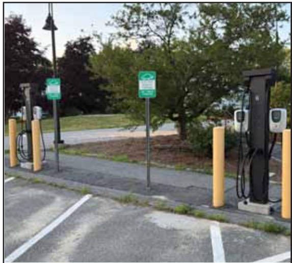
CHARGING STATIONS GEORGETOWN PEABODY LIBRARY No bids, managed by Town Admin. Orlando Pacheco. Required changes. Contractor: Inovis TOTAL PROJECT COST: $103,672
