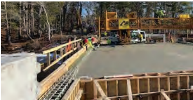
The deck for the bridge was poured in December (Photo provided by the town of West Newbury)
