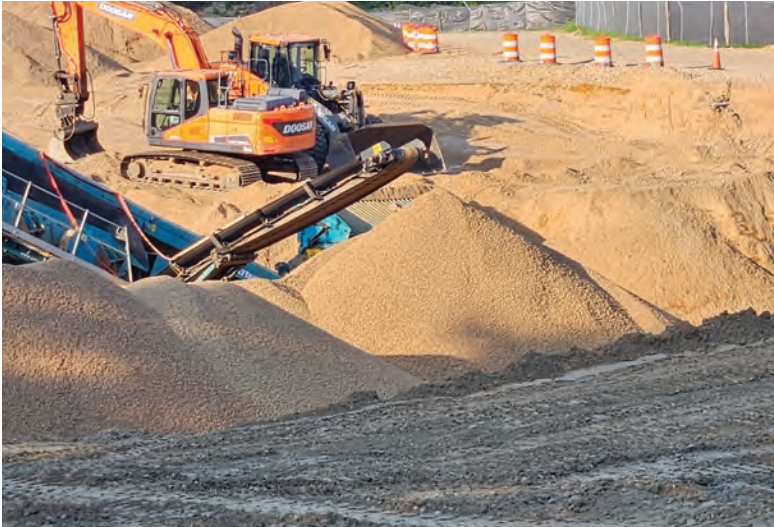
Conveyor hauls sand up from the 19' deep sand mining operation. - August 2025
