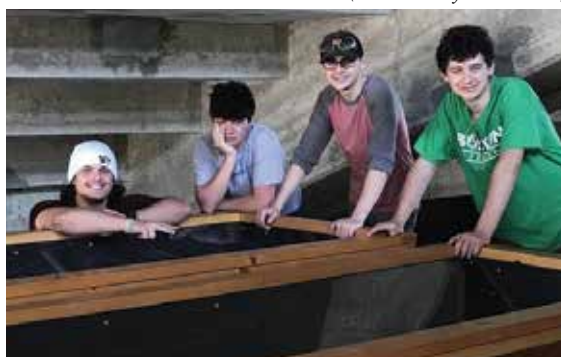
From left, William King, Christopher Bognanno, Noah Gayner, and Craig Kielbania stand with the completed garden beds built for Haverhill Brightside, Team Haverhill, and Haverhill Garden Club. (Photo Courtesy Whittier Tech)
